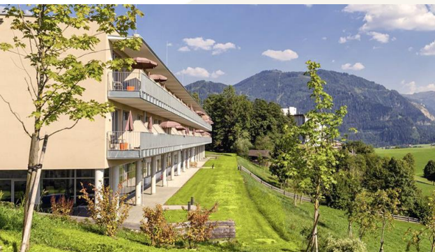
Onkologische Rehabilitation St. Veit, 120 Betten
